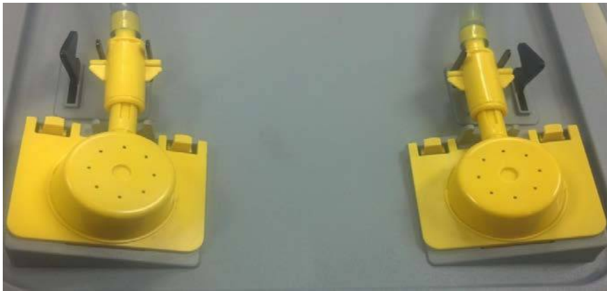
Figure 2: Nozzle Assemblies installed
